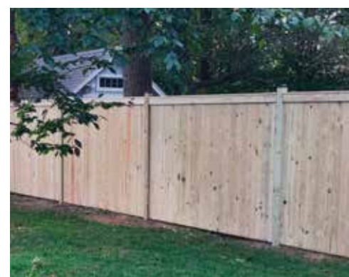
Vertical Board - Cap and Fascia
